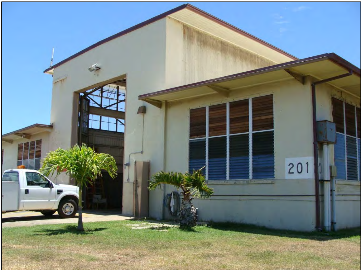
Enclosure 15. Facility 201, front view, showing that the shape and overall massing of the building has remained the same.
