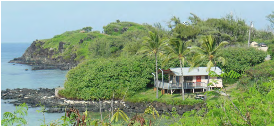
Oblique view of Existing Cottage 1612
