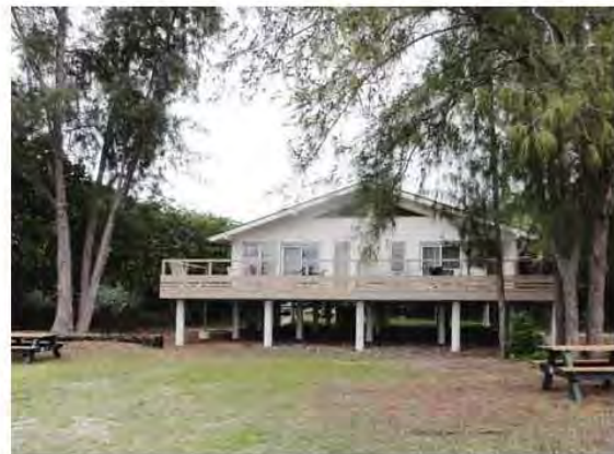
Photo of Existing Duplex Cottage (6171)
