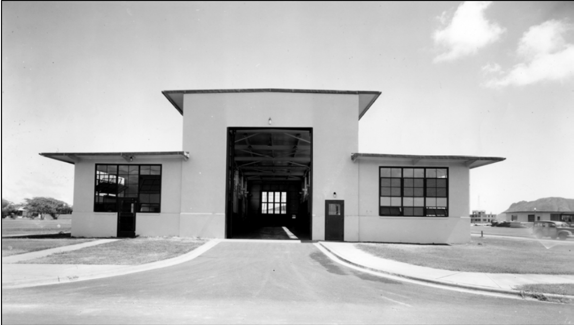
Enclosure 14. Utilities Shop and Parachute Loft-Stowage building constructed 1941 (photo dated 9 Sept 1941).
