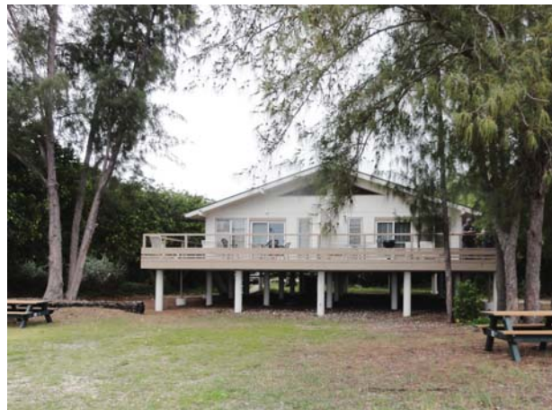
Photo of Existing Duplex Cottage (6171)
